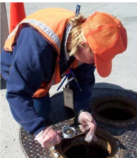
District Compliance inspectors make sure vapor recovery systems are working both at the pump and at the underground storage tank.
