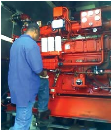
A District mechanical engineer records engine operating data in support of a source test.
