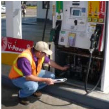
District inspectors ensure that vapor recovery equipment works properly.
