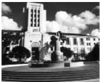
San Diego County Administration Center
