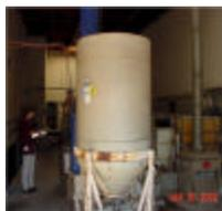
This cone-type waste treatment tank is typically used to allow for toxic metals to settle to the bottom of the tanks, while the liquid waste stays on top. A sludge waste is generated. The liquid waste may be treated again depending on the circumstances.
