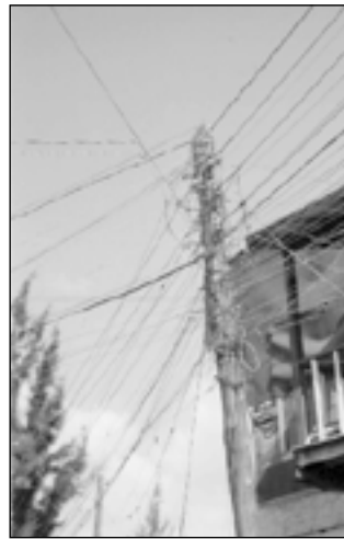
Informally tapped electricity in maquiladora workers’ community in Tijuana.
