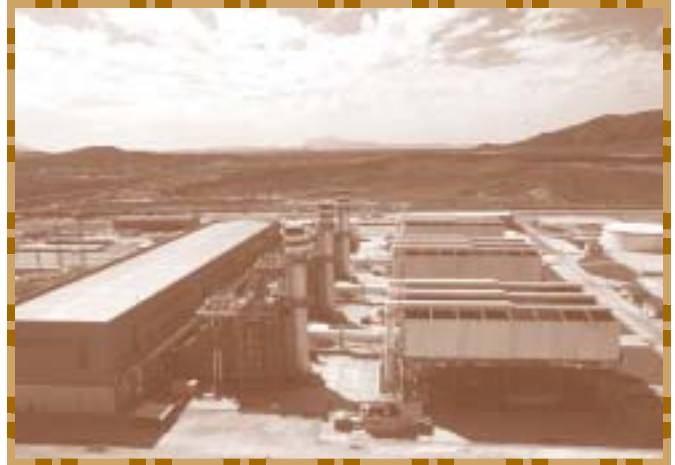
This Samalayuca combined-cycle power plant near Ciudad Juarez, Chihuahua, and El Paso, Texas, uses air cooled condensers. Photo credit: GEA Power Cooling Systems.
